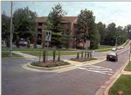
Additional example of roadway narrowing
