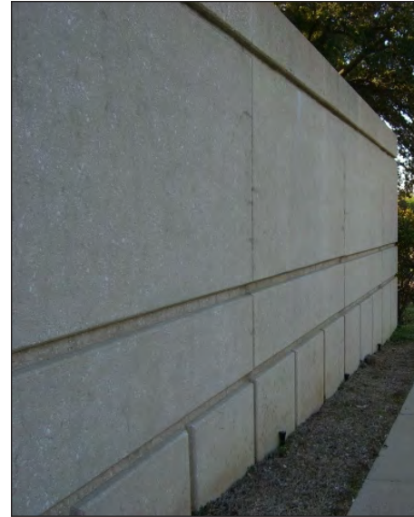
Retaining walls frame existing landscaping
