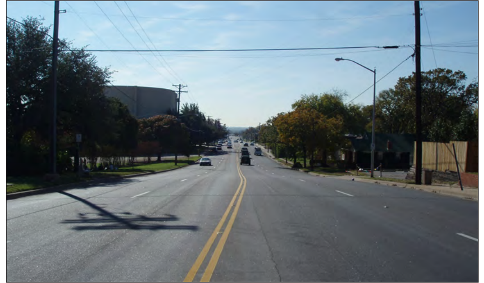
Montgomery and Tulsa Way - Looking North
